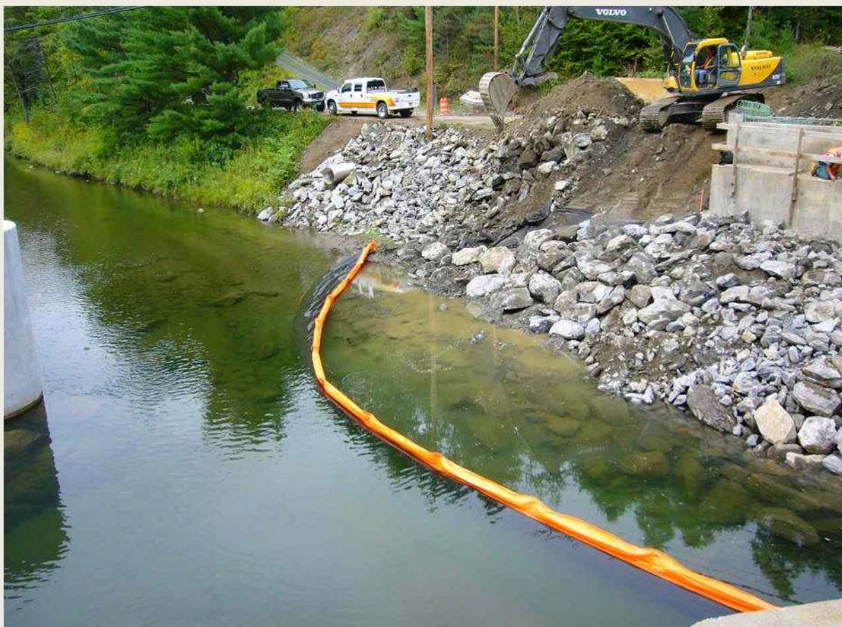
Filter curtain at work Rt. 110 Tunbridge, VT
