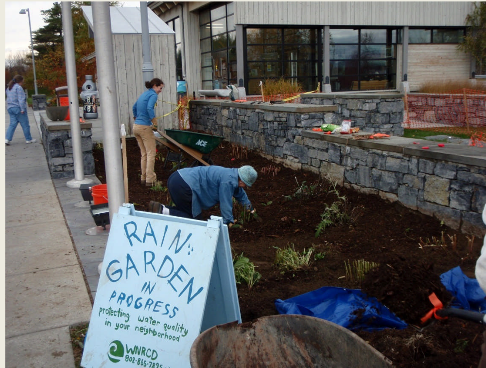
Williston I-89 NB Welcome Center Rain Garden Installation
